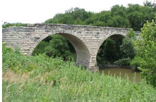
An Arch Bridge in Clements, Kansas
