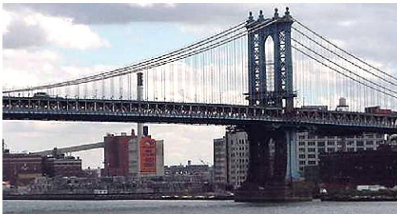
'M' Shape Bridge in New York City
