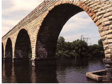
An Arch Bridge in Minnesota
